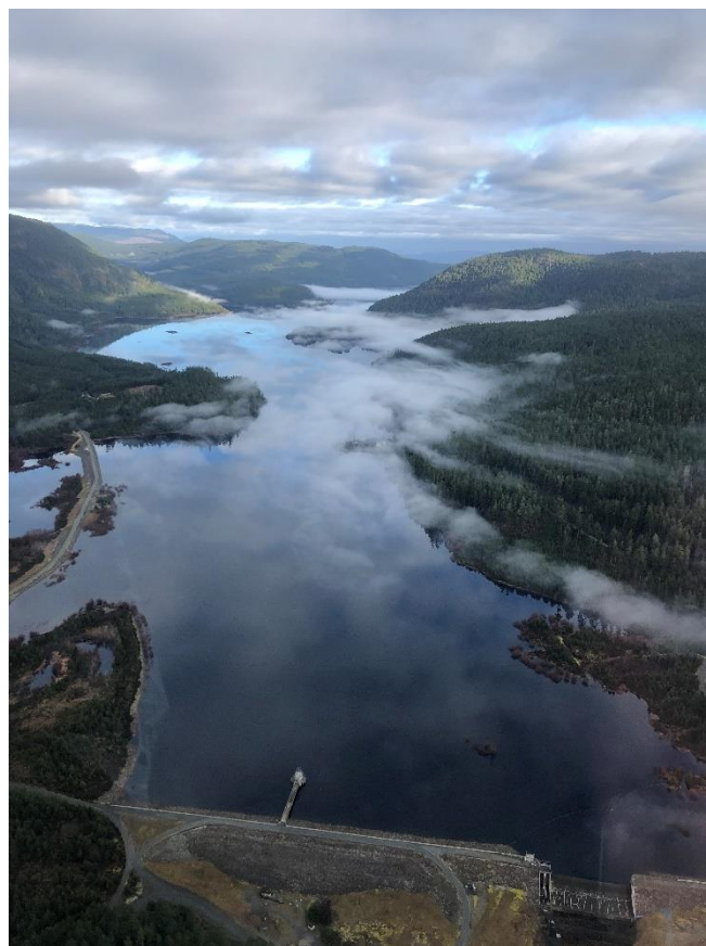
Photo of the Sooke Lake Reservoir
